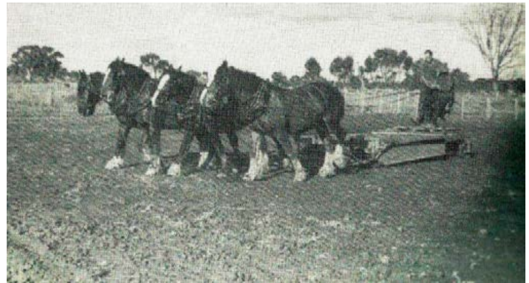
Soil grading with a 'Harvey' box grader—July 1937.
